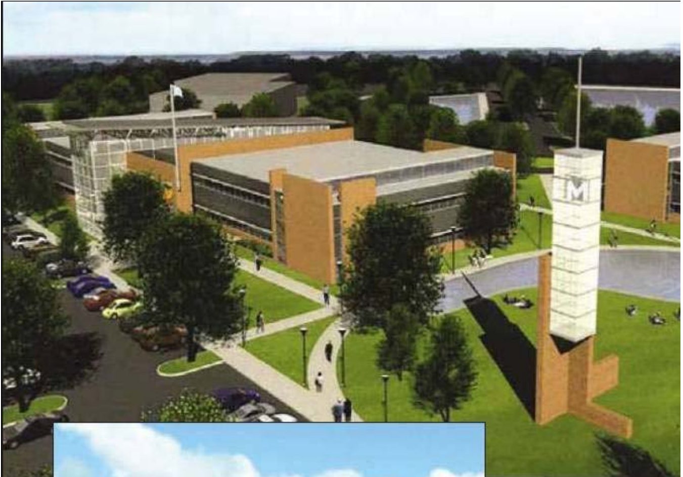
RENDERINGS COURTESY OF THE CITY OF SUFFOLK The 32-acre lot chosen as the new site for the Virginia Modeling, Analysis and Simulation Center straddles Suffolk and Portsmouth.
